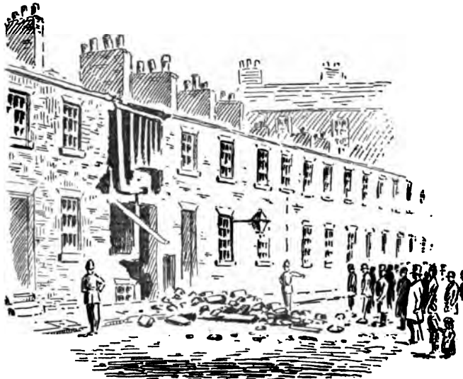
Effects of Explosion in Ellison Terrace.
